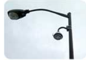
Double duty – Another view of a Sony SNC-RZ30N mounted high up in a light pole shows how authority staff used existing infrastructure.
