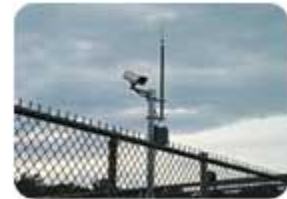
Looking inward — Sony SNC-Z20N fixed-focus camera mounted in an Everfocus outdoor housing with heater strip and blower.
