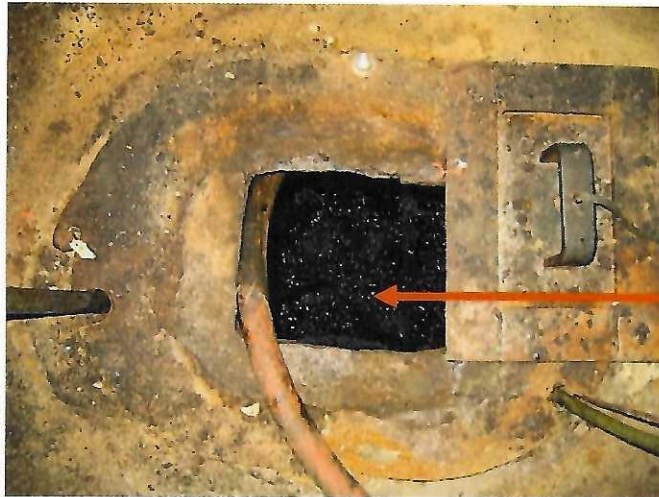
Sampling Point: Located in Sewer Room in Building
